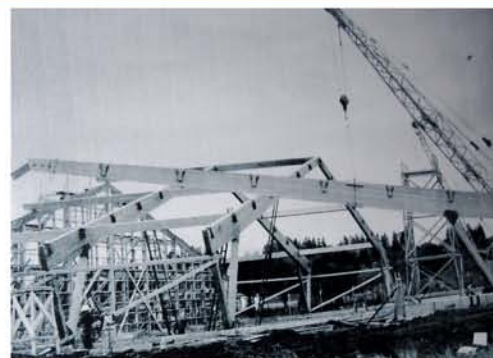
Rink Under Construction
